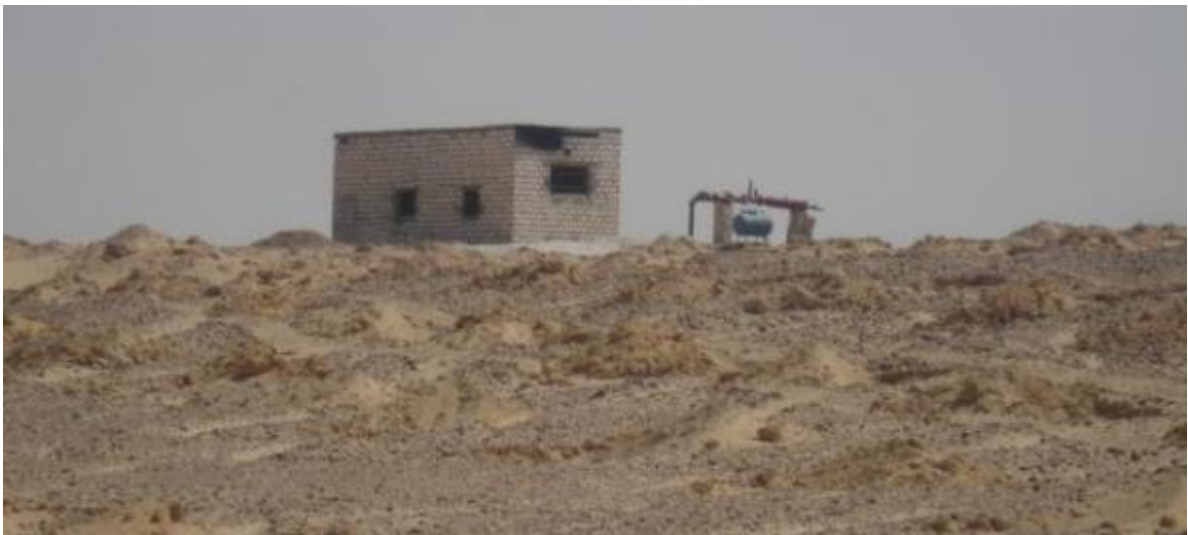
Water well ( Al-Hag Alaa Farm )
