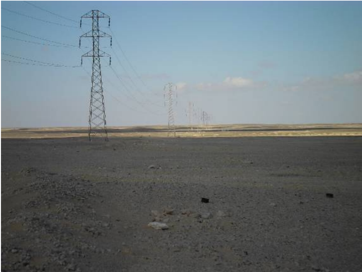
Intersection paved road in Over head transmission line track at the area 28 22 43.7 N 30 19 29.78 E
