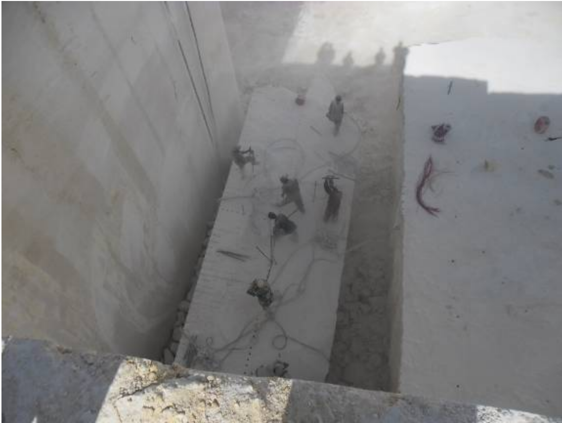
Labor +Activities at Crusher and marble area in North side of the area 28 29 57.1 N 30 15 8.4
