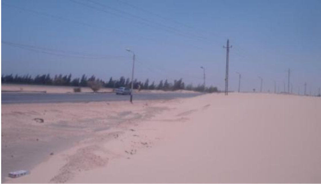
Sand dune encroaching the main road
