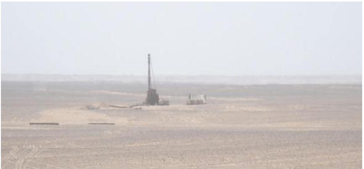
Groundwater drilling Machine ( Rig )
