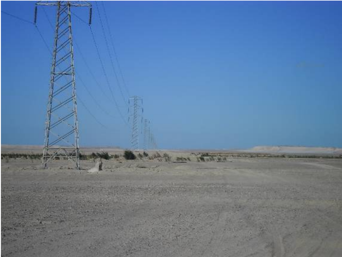
Hilly mountain in Over head transmission line track at the area 28 19 25.7 N 30 27 36.78 E
