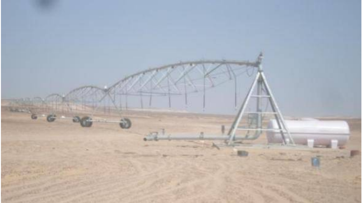
Irrigation System ( Pivot ) under construction , area under reclamation
